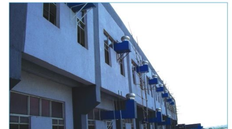
Installation on side wall
