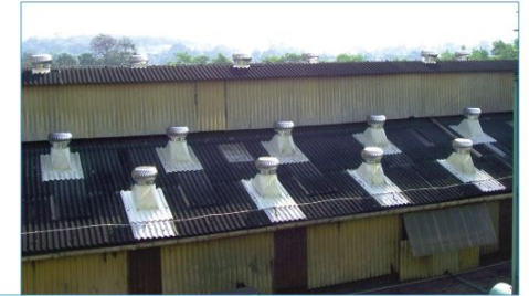
Installation on shed with fully corrugated asbestos roof sheet
