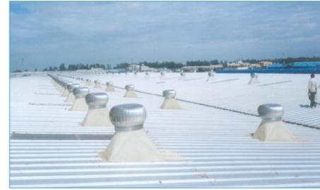
Installation in prefab shed with colour coated metal sheet
